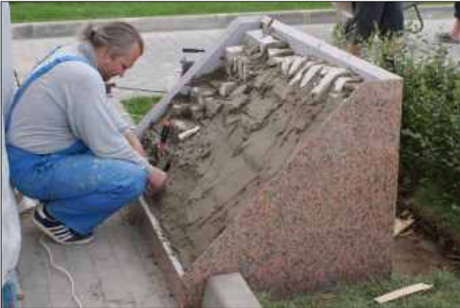
Fig. 7. Rubble infill of the information plate stand.
